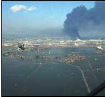
Helicopter view of Sendai, Japan after 2011 tsunami which shows damage in the Tōhoku region with black smoke coming from the Nippon Oil Sendai oil refinery
