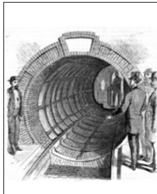
Entrance pneumatic transit
